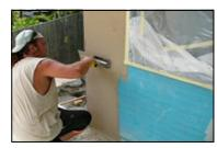
Top Picture: Alfresco Graincoat tinted Bottom Picture: Alfresco Medium Sand applied by steel trowel in preparation to be over-coated with Alfresco Graincoat. Both can be tinted to almost any colour and comes in 15 litre pails.
